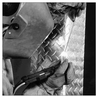
Figure 8.9 Welding in the vertical position.
